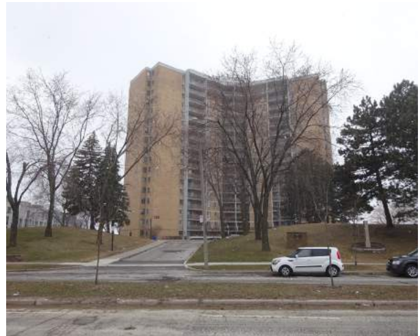
120 Widdicombe Hill Boulevard, View looking west
