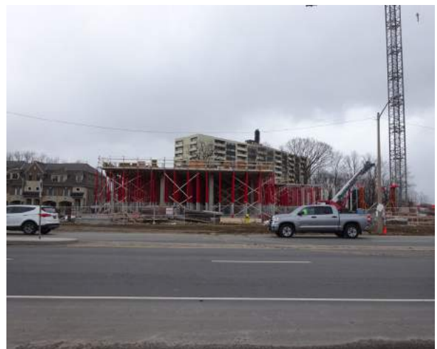
4650 Eglinton Avenue West, View looking north
