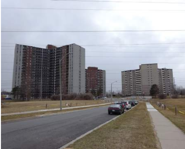
22, 36 and 44 Willowridge Road, View looking west along Richgrove Drive
