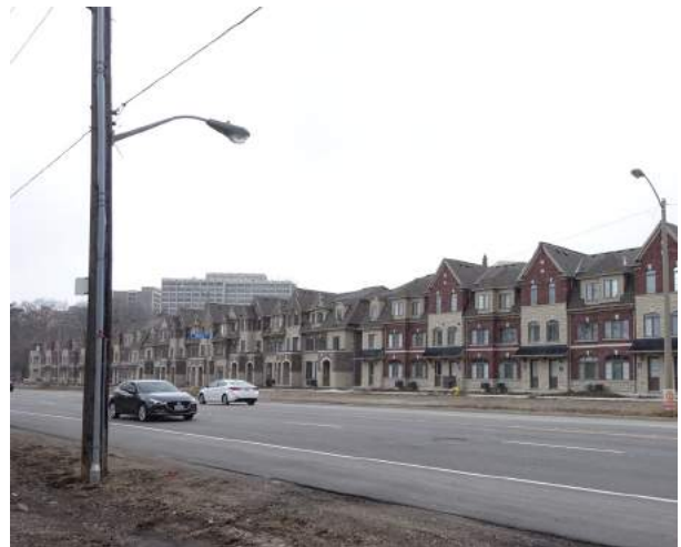
9 to 76 Dryden Way, View looking northwest
