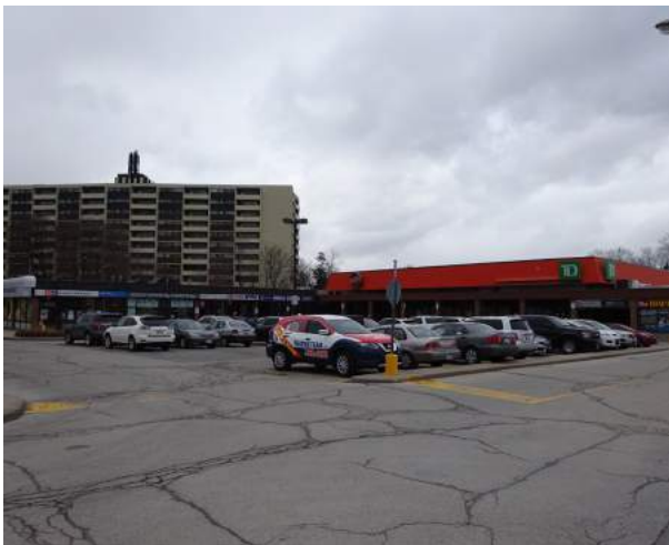
Subject Site, Existing Plaza, View looking northwest
