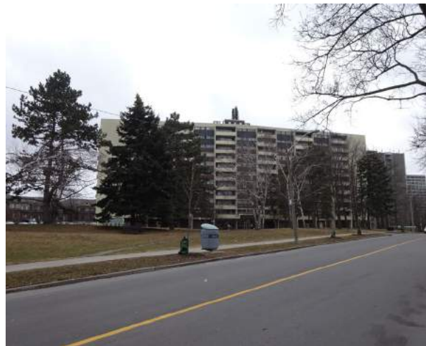
35 Widdicombe Hill, View looking southwest
